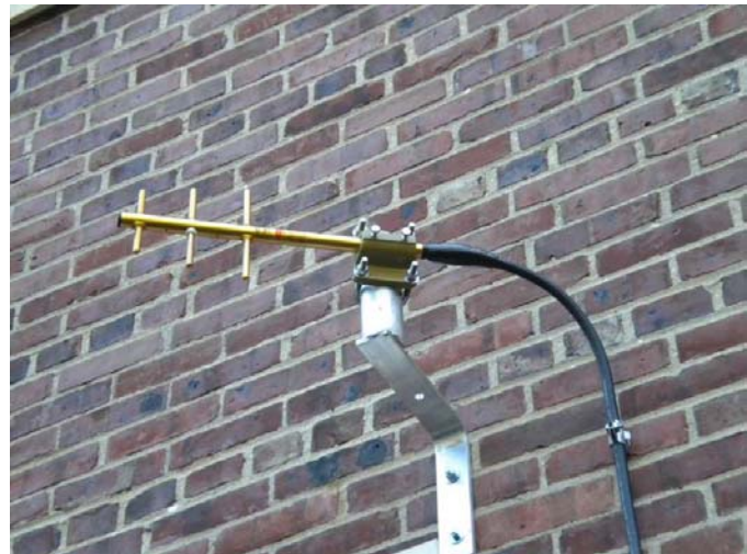
Wall Mount installation (Standard Model)
