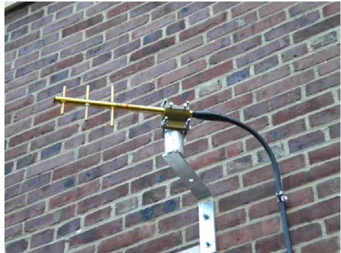
Wall Mount installation (Standard Model)
